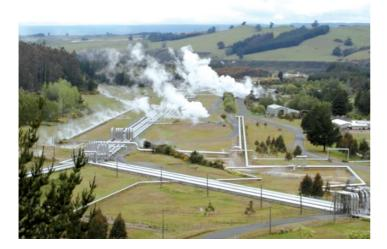
Hot rock under the surface of the earth can heat water converting it to steam. This then generates electricity in the same way as coal, oil, gas or nuclear powered stations.
